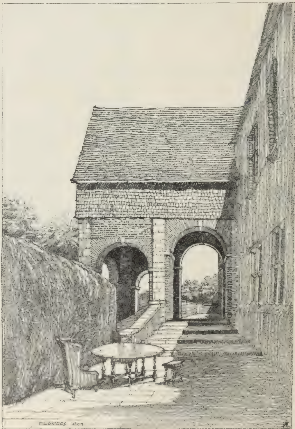
A PORCH AND TERRACE
